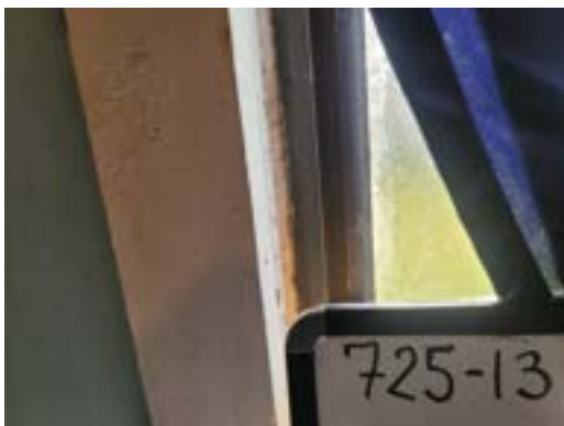
725-13 Caulk Typical Interior Windows
