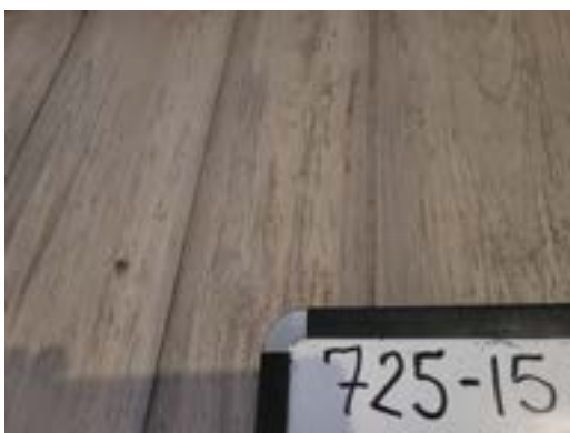
725-15 Paneling Laminate Interior Utility Porch Walls
