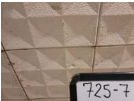
725-7 12"x12" Ceiling Tile Interior Living Room
