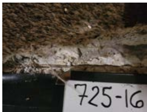
725-16 Floor Leveling Compound Interior NE Bedroom
