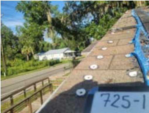
725-1 Asphalt Shingle/Tar Typical Exterior Roof
