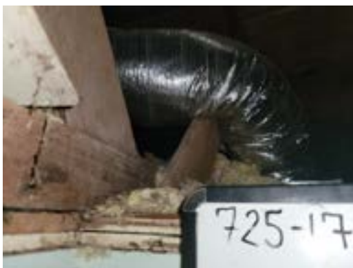
725-17 Insulation Interior Attic Crawlspace
