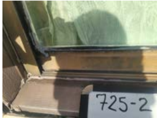
725-2 Caulk Typical Exterior Windows
