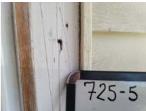
725-5 Caulk Exterior Front Door
